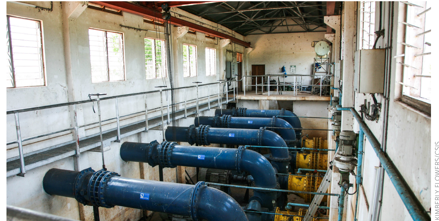
The irrigation pumps at Dakawa currently break down twice a week for six to 12 hours at a time. Feed the Future plans to rehabilitate this pump house, which serves hundreds of rice farmers in the area.
